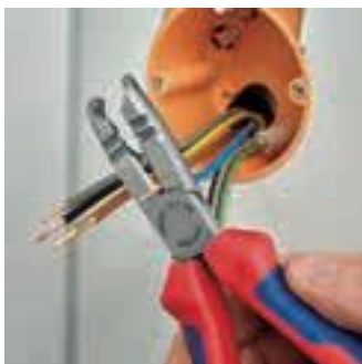
Cutting when shortening single conductors
